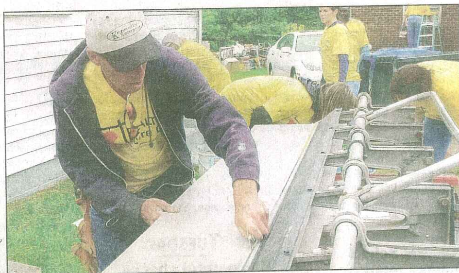
Chris Tese , an employee of Kennedy Enterprise in Mooresville, cuts metal for repairs to the siding and eaves of one of the homes.
